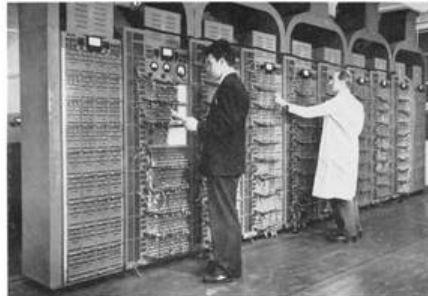
Plate 13 (a). Analogue computer system designed by E.M.I. Electronics as a simulator for studying complex control problems associated with guided weapons.
