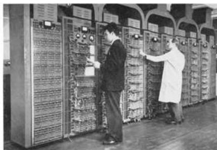
Plate 13 (a). Analogue computer system designed by E.M.I.
